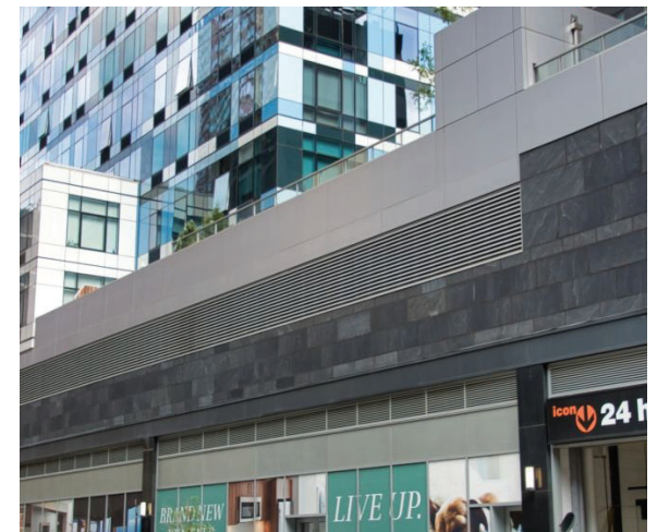
Figure 63: Jay St Metro Tech Station, New York Courtesy of Nicolas Janberg and structurae
