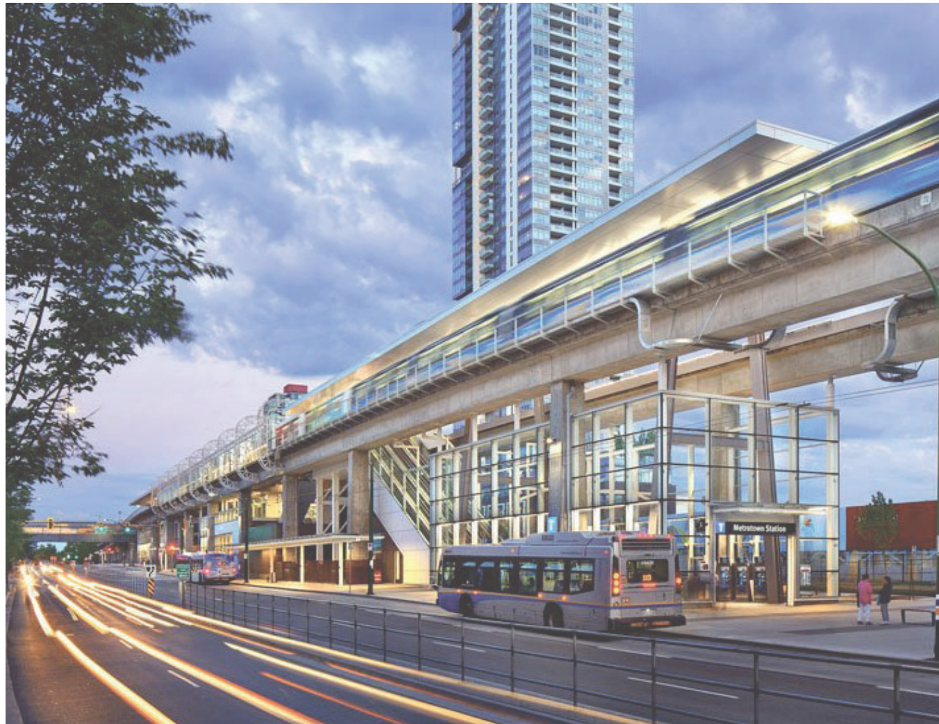
Figure 8: Metrotown SkyTrain Station, Burnaby Courtesy of https://canada.constructconnect.com
