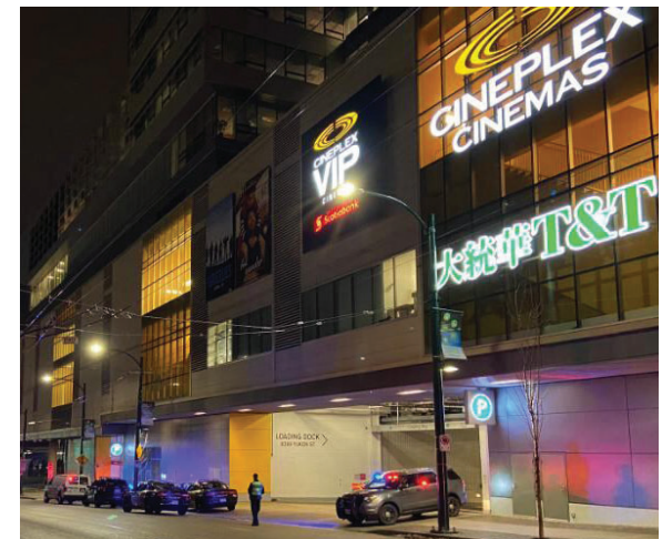
Figure 65: Service Access, Marine Gateway, Vancouver Courtesy of https://www.cbc.ca
