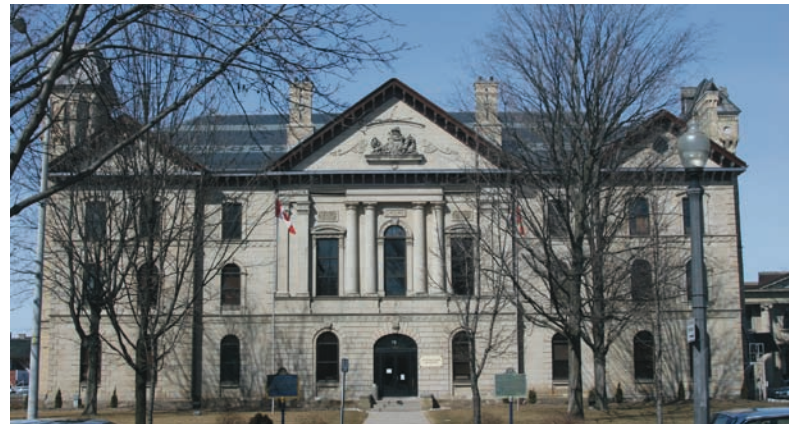
Brant County Courthouse – 70 Wellington Street, Brantford
